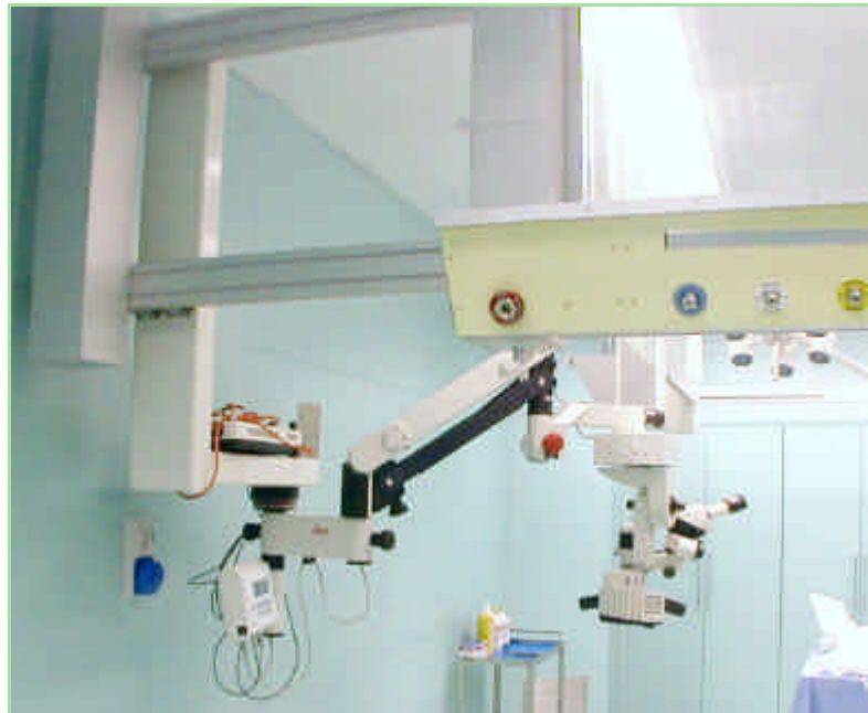
Operating theater „Casa di cura Villa Chiara“ in Casalecchio di Reno. Option of heavy arm specifically designed to carry microscopes.
